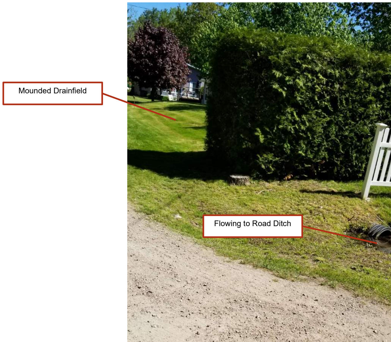
Another example of mounded drainfield with a direct discharge to road ditch under it.
